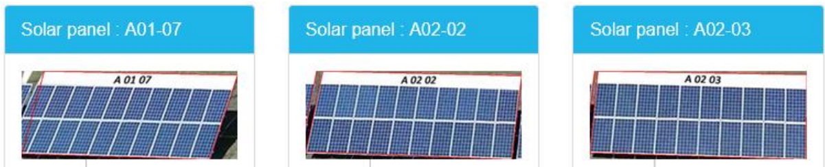
Figure 5.11 System screen - Solar panel label identification
