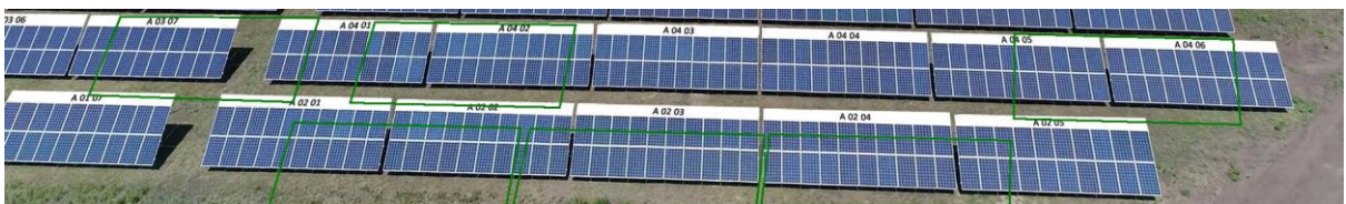
Figure 5.8 System screen - Wrongly marked solar panels edges
