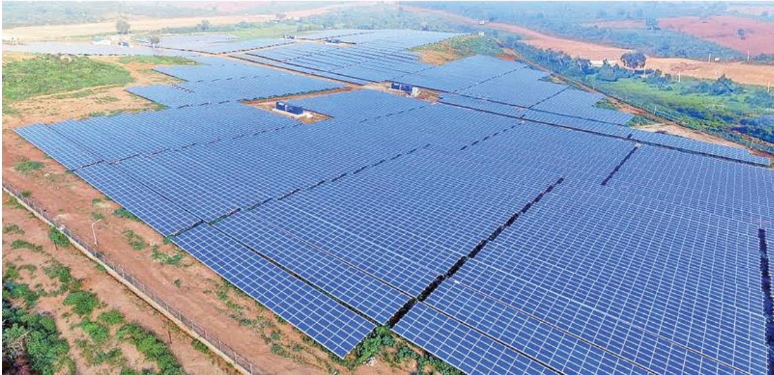
Figure 3.2 Solar power station
